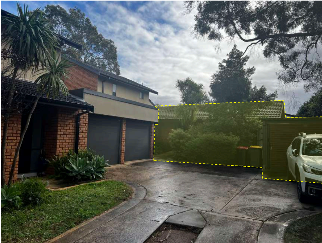
Figure 3. The site (Unit 1 highlighted)
